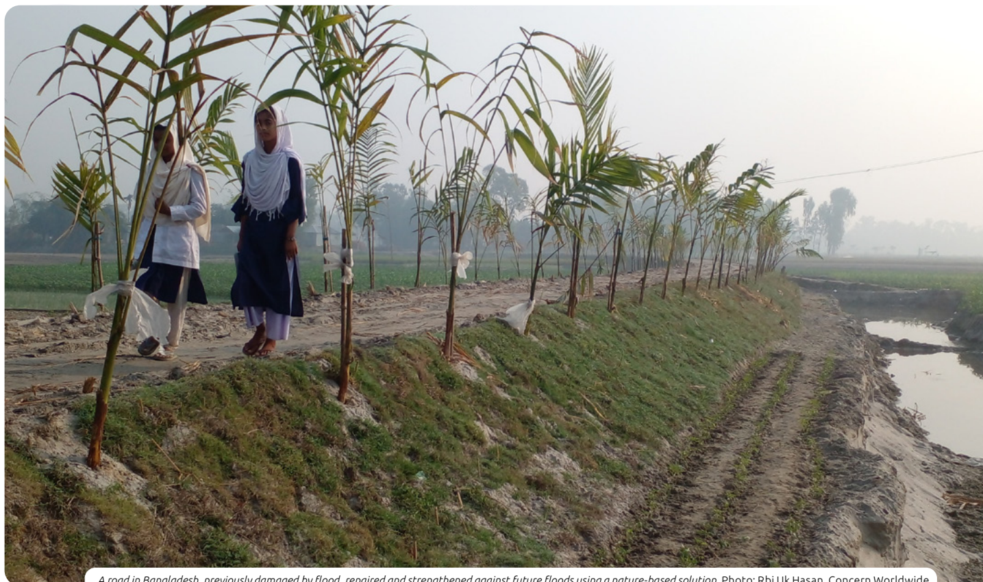
A road in Bangladesh, previously damaged by flood, repaired and strengthened against future floods using a nature-based solution. Photo: Rbi Uk Hasan, Concern Worldwide
