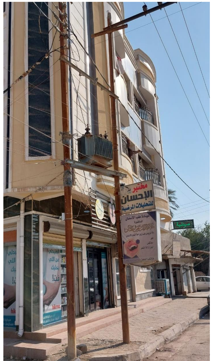
No circuit breakers, No Link Fuse, No Earthing, Rusted poles
