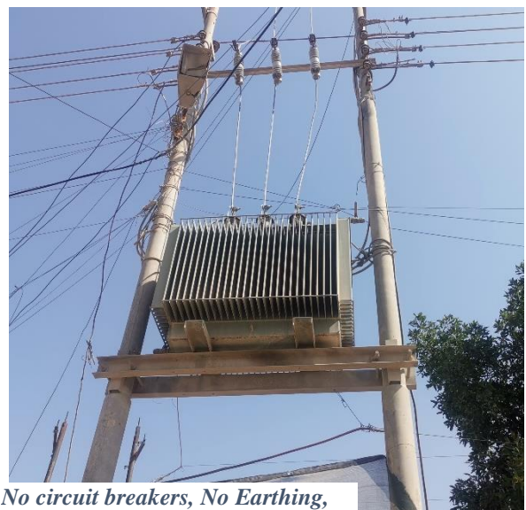
No circuit breakers, No Link Fuse, No Earthing, Rusted poles
