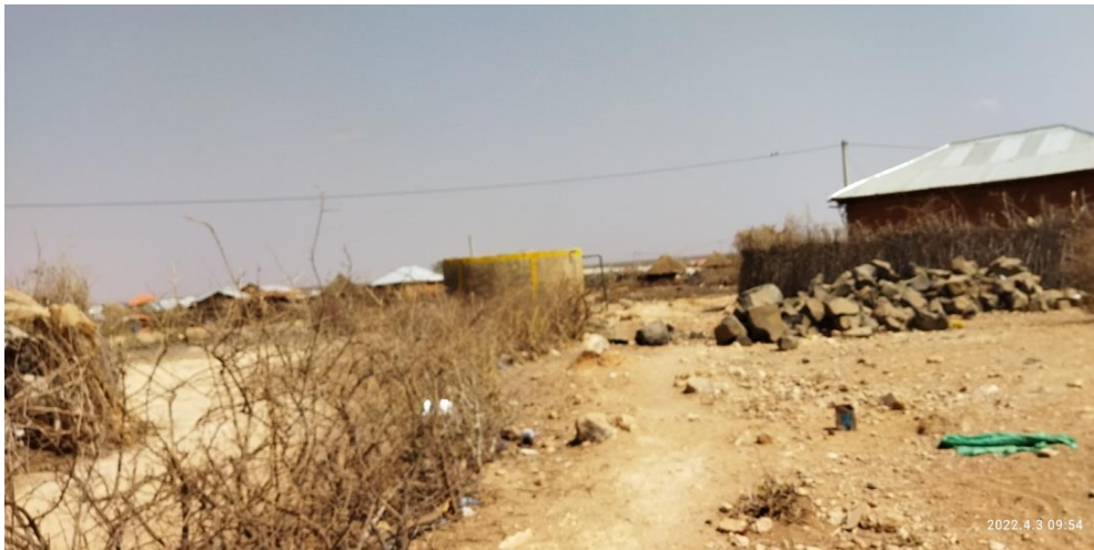
Figure 4-6 50m 3 service reservoirs
