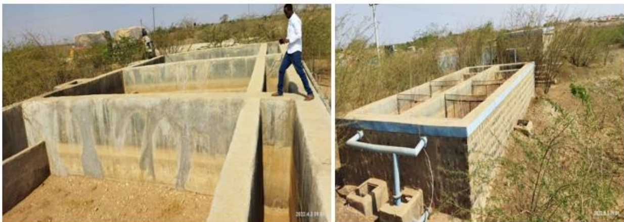
Figure 4-2 Sedimentation Tank with horizontal clarification
