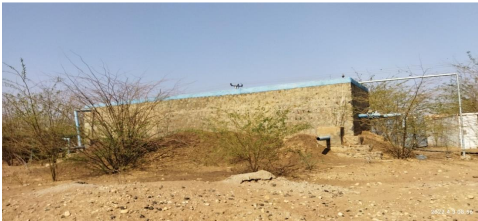
Figure 4-4 Rectangular raw water Collector Tank
