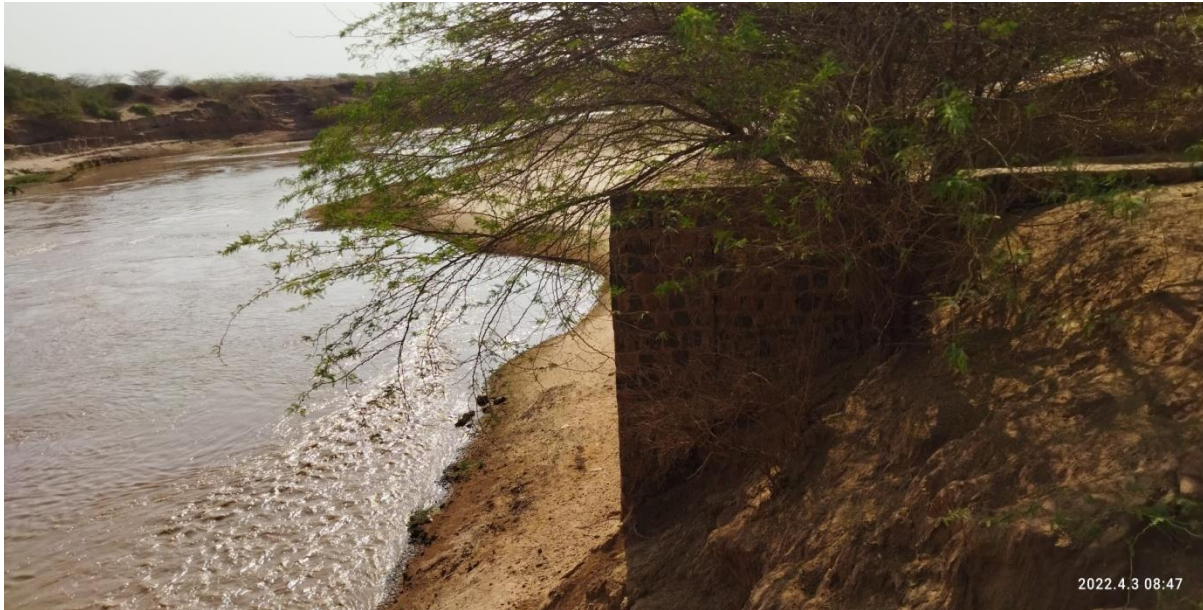
Figure 4-1 River intake structure
