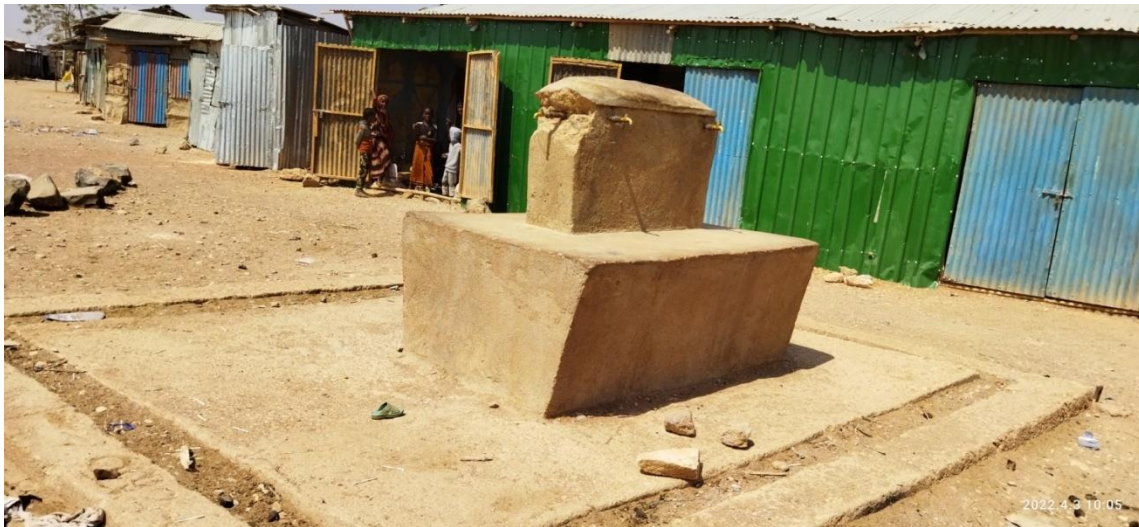
Figure 4-8 Public water point in Adadle
