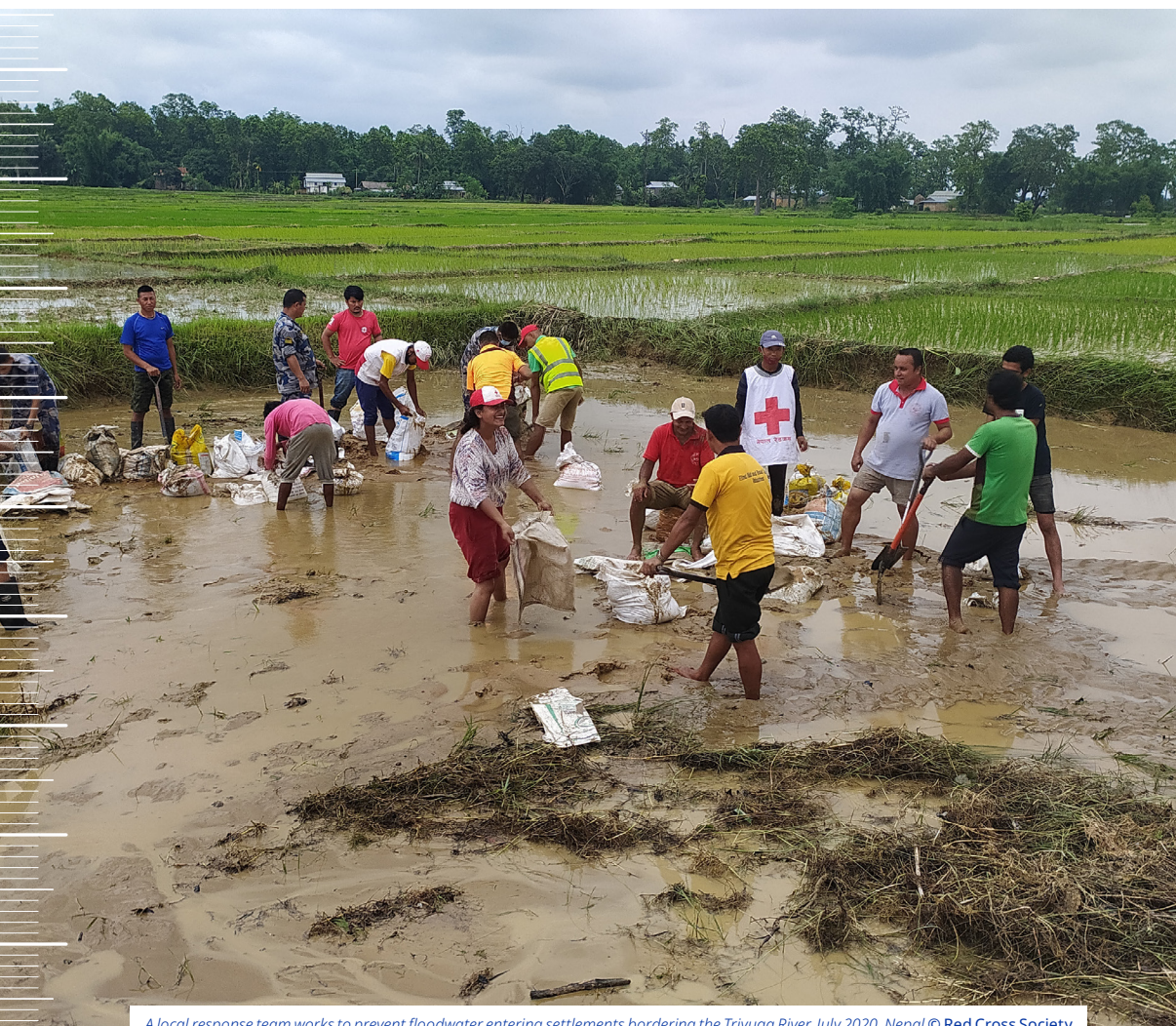
A local response team works to prevent floodwater entering settlements bordering the Triyuga River, July 2020. Nepal © Red Cross Society
