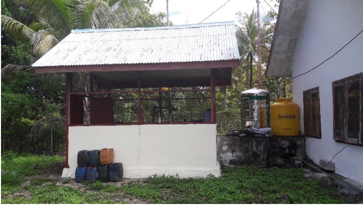
Figure 3: Existing diesel generator housing shed
