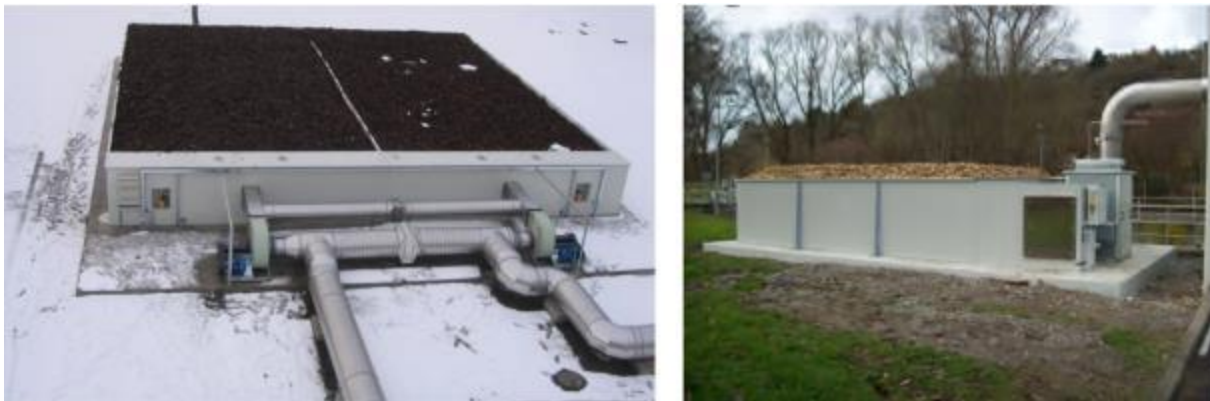
Figure 12 : Typical Biofilter
