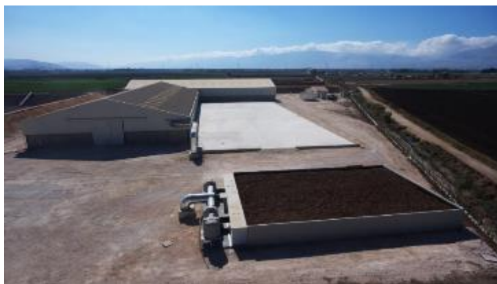
Figure 13 : Biofilter in Bar Elias designed by Libanconsult AGM within a similar study
